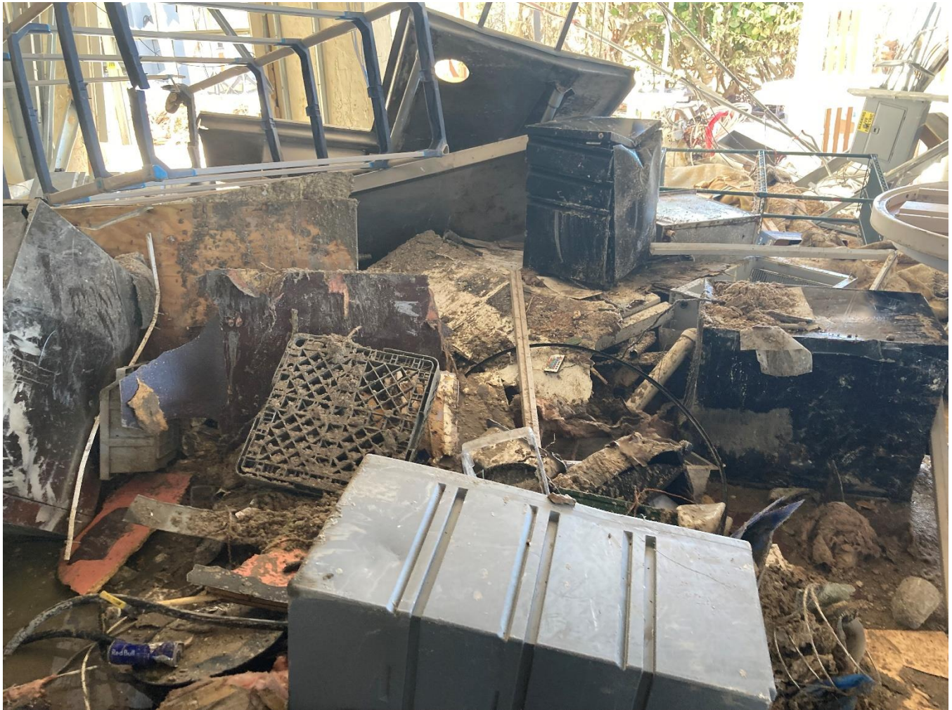
Damage to restaurant in Vanderbilt Beach caused by storm surge from Hurricane Ian (NWS Storm Survey picture)
